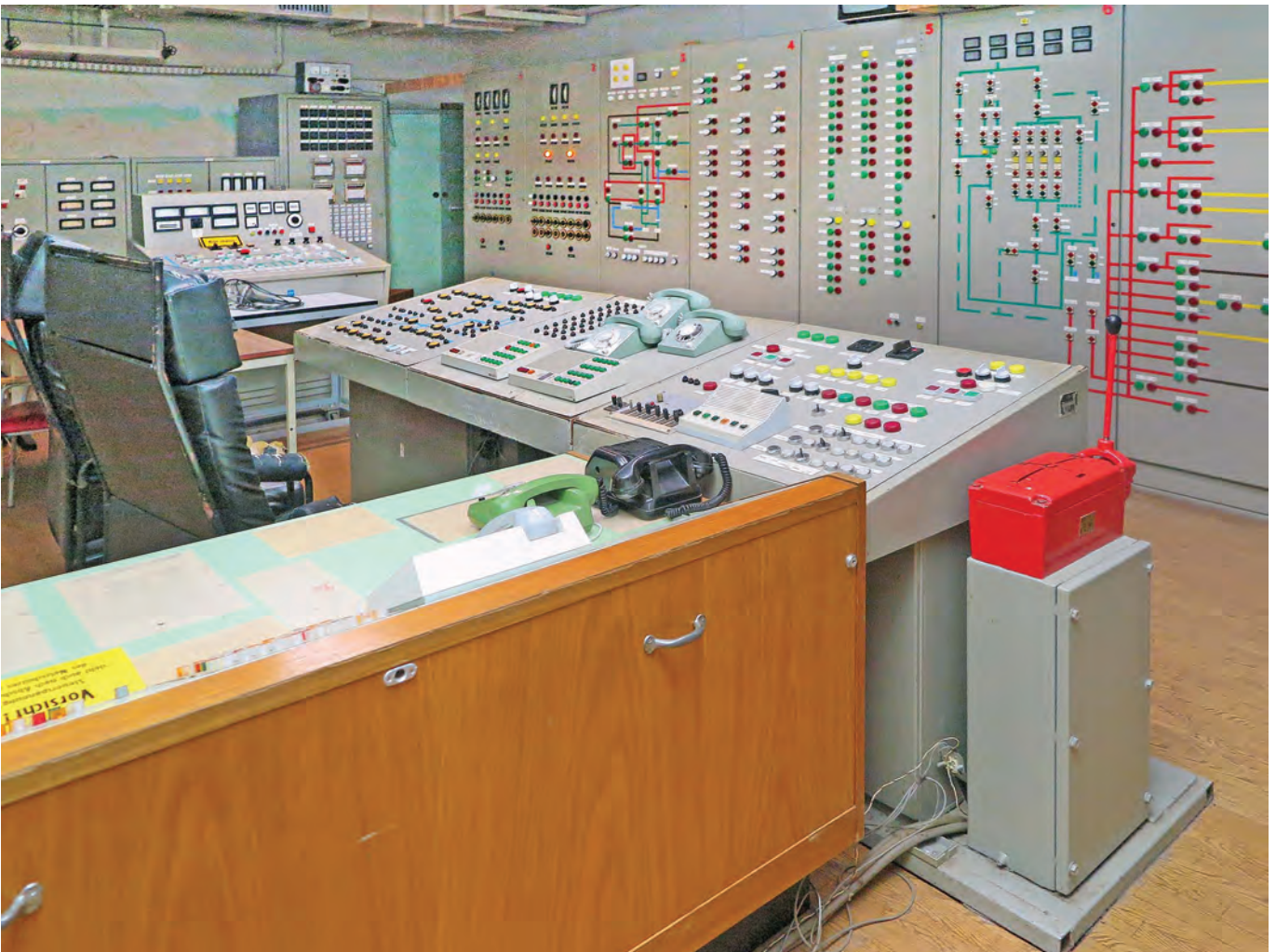
Harnepok bunker dispatch room, the red lever being to switch between bunker readiness modes. Photo Clive Penfold
